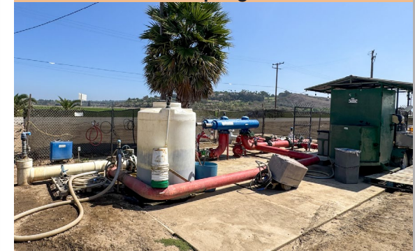
Main Pumping Station
